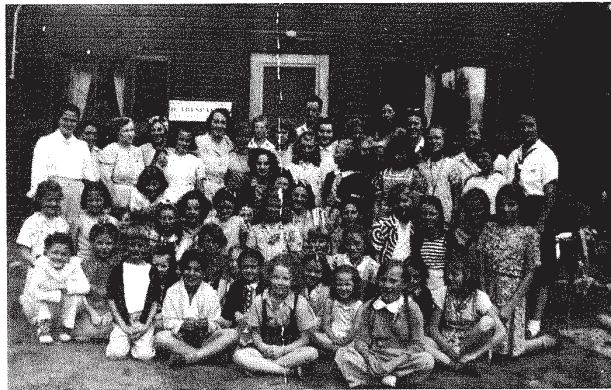
Main Lodge Completed 1942
